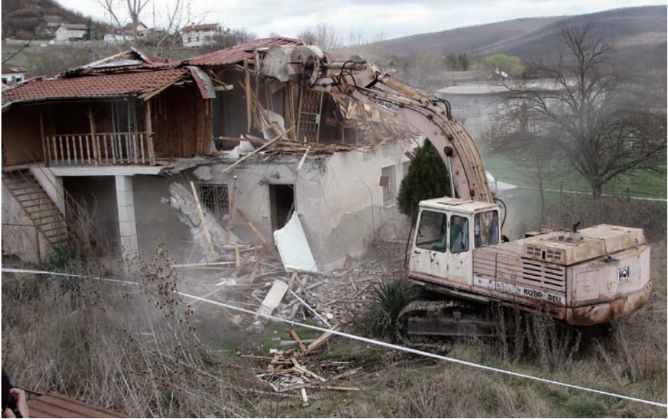
Figure 13. Bulgaria: Demolition of informal construction
