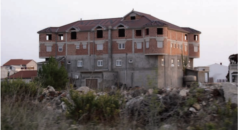
Figure 12. Croatia: Informal construction intended for commercial use in Vir settlement
