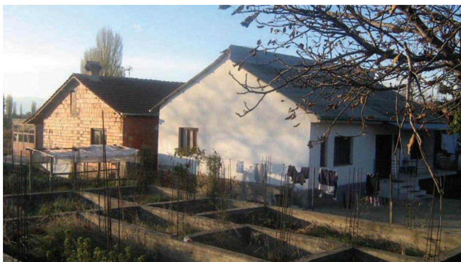
Figure 17. Macedonia: Prilep – modest individual houses in the informal settlement
